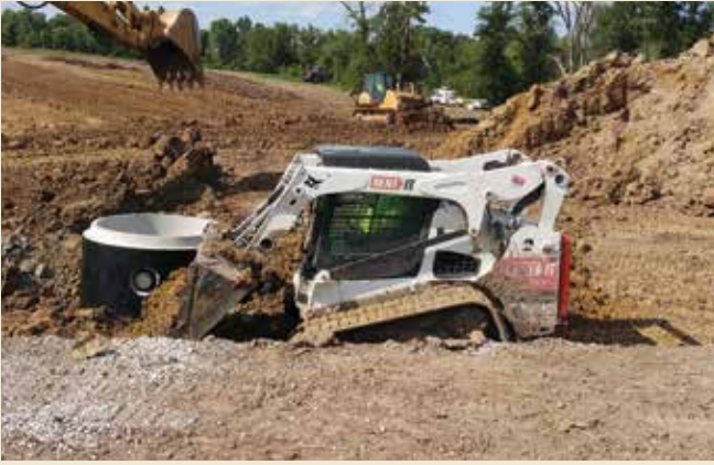
Bobcat of Columbia's skid steer helps to backfill the wet well.
