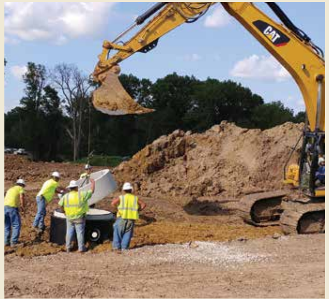
Contractors lower the last section of the wet well into place.
