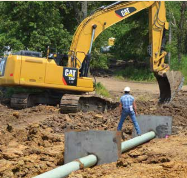
Kevin Waller watches as water-packing the spillway begins.
